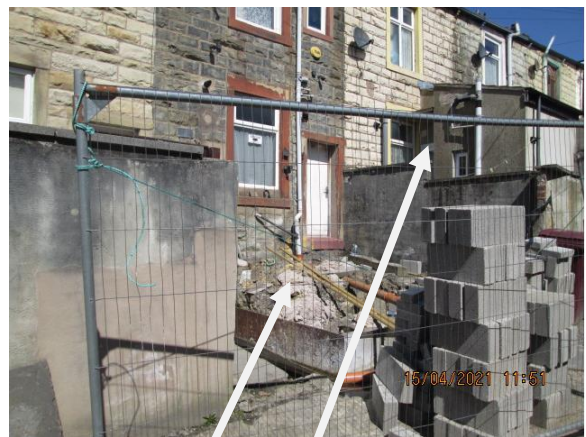
rear of 87 and 89 Brougham Street
